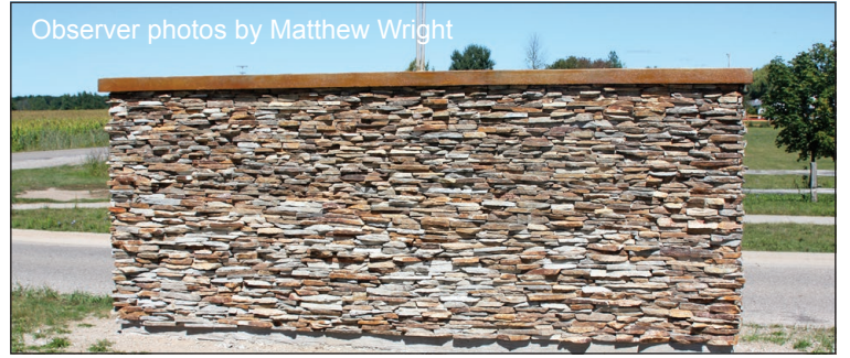
After: Scenic stonework hides the graffiti vandalism.
