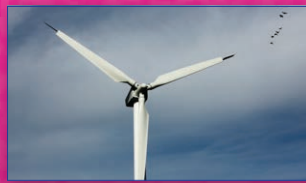
Wind Turbine off Tomah Road
